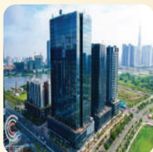
The Crest Residence
